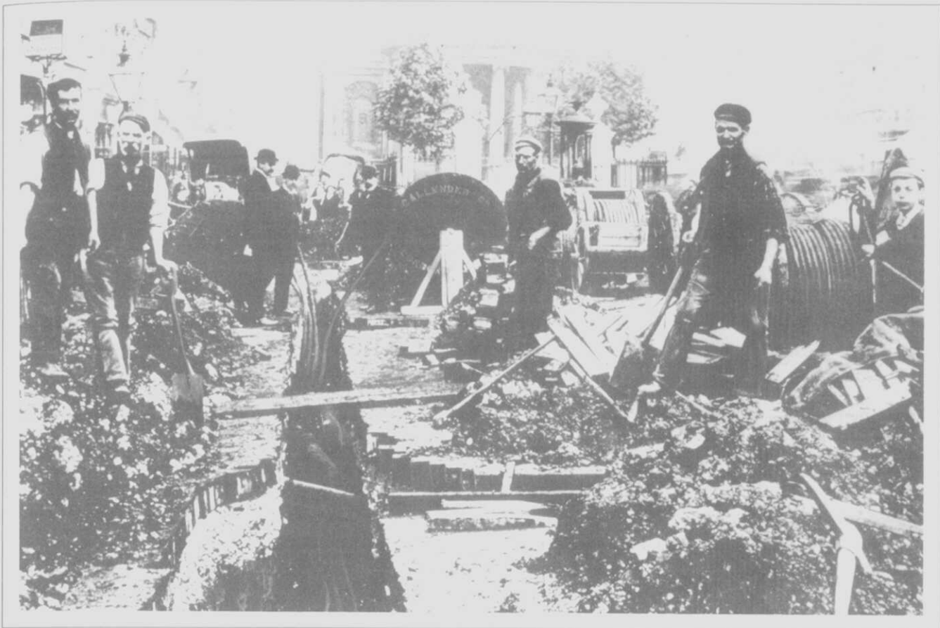
Plate 9 Cable laying in The Strand by St Clement Danes, 1895. (Courtesy B.I.C.C.)
